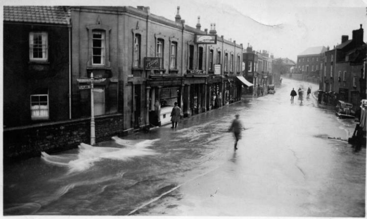
Fig 3. Westbury-on-Trym Flooding, c1938
