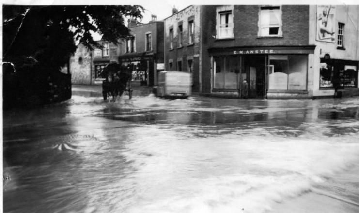
Fig 5. Westbury-on-Trym Flooding, c1938
