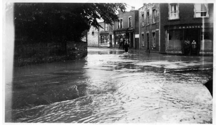
Fig 4. Westbury-on-Trym Flooding, c1938
