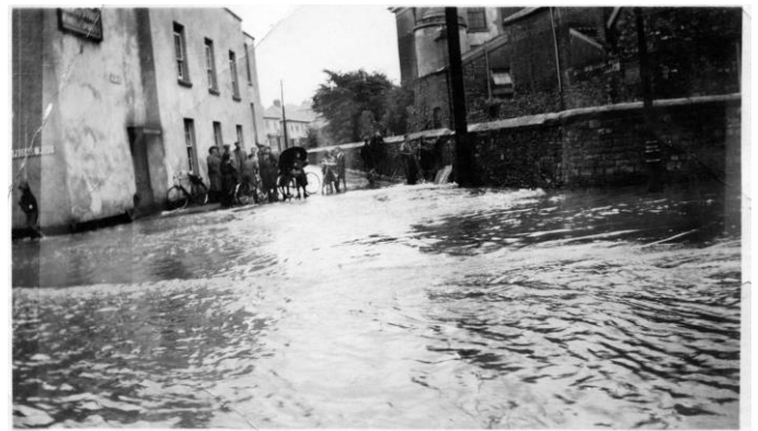
Fig 6. Westbury-on-Trym Flooding, c1938
