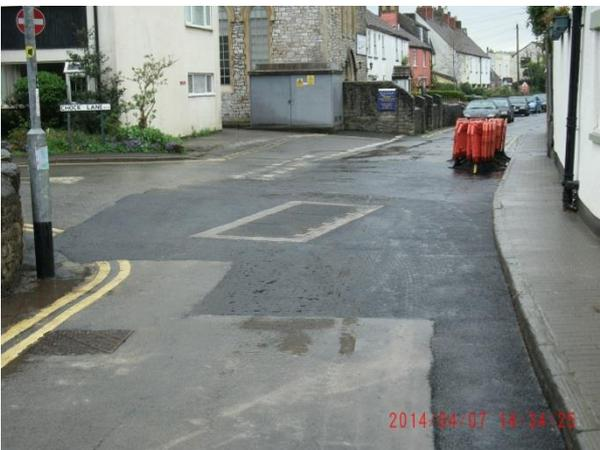
Fig 7. New chamber cover – fully fitted
