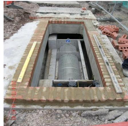
Fig 6. New chamber – topped out
