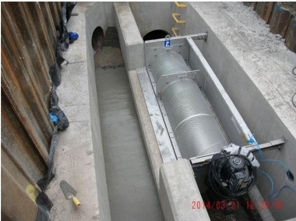
Fig 5. Rotating screen in position
