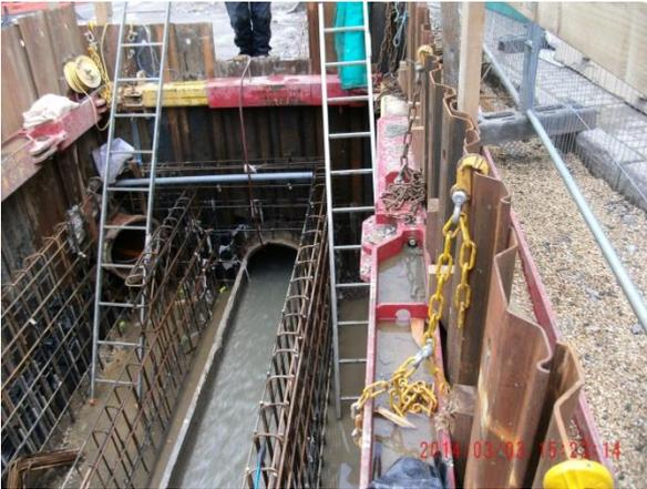
Fig 3. New chamber, partially constructed
