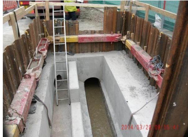
Fig 4. New chamber with new weir
