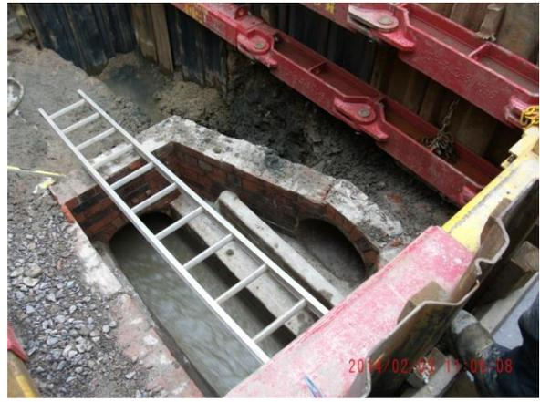
Fig 2. Fixed overflow weir in original chamber
